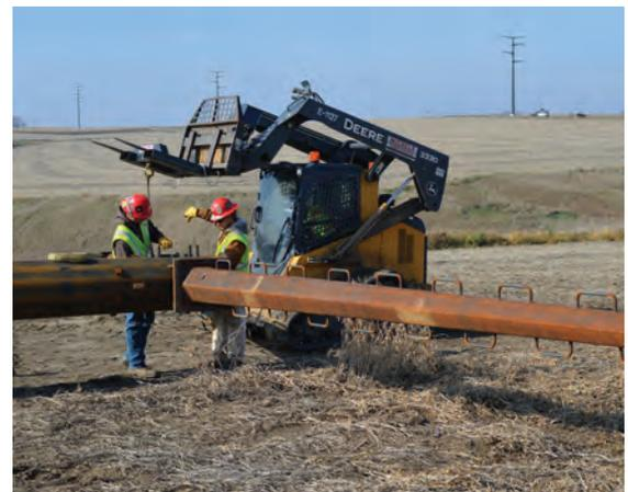
*Crews frame a structure prior to setting it near White, S.D. Structures on the Big Stone South-Brookings County project are between 140-170 feet tall and are typically about 1,000 feet apart.*
