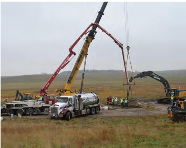
*The last foundation is poured on the Big Stone South-Brookings County project. More than 33,000 cubic yards of concrete were used to construct project foundations.*
